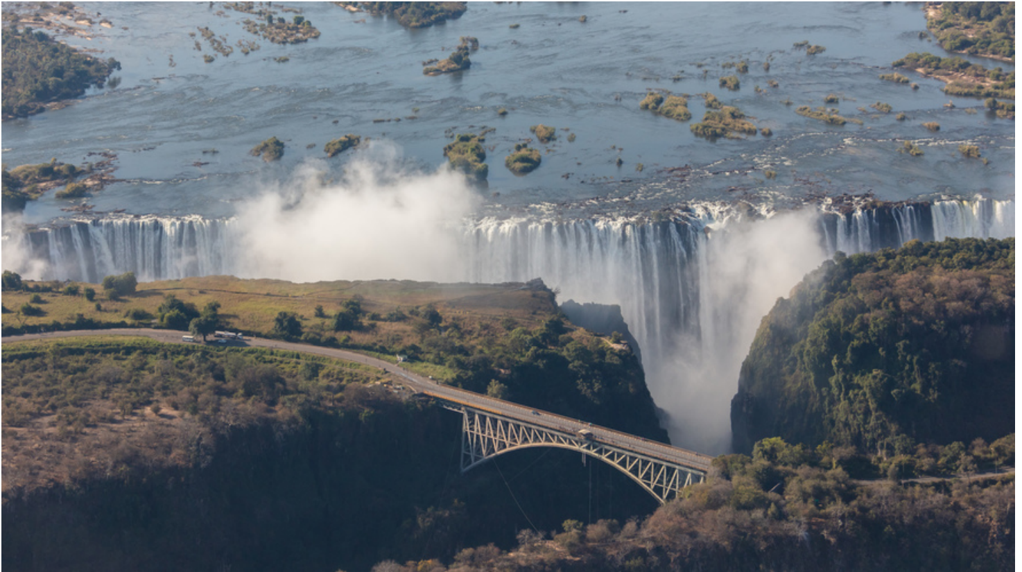
Image 1. The bridge over the Zambezi River at Victoria Falls separates the countries of Zimbabwe and Zambia. Photo by Diego Delso, delso.photo, License CC-BY-SA via Wikimedia Commons.
